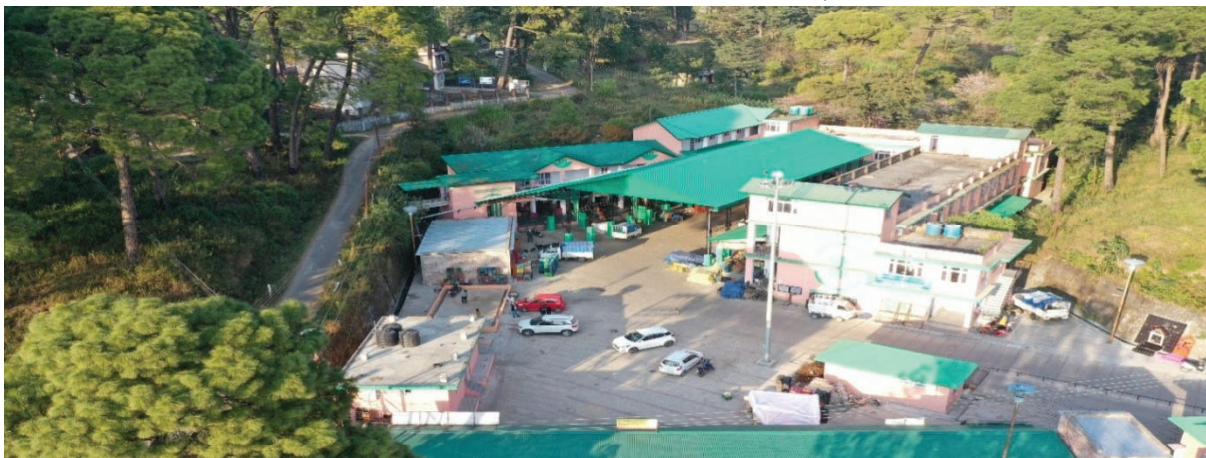
FIG 2 Photograph of Kangni Market Yard (Work Completed)
